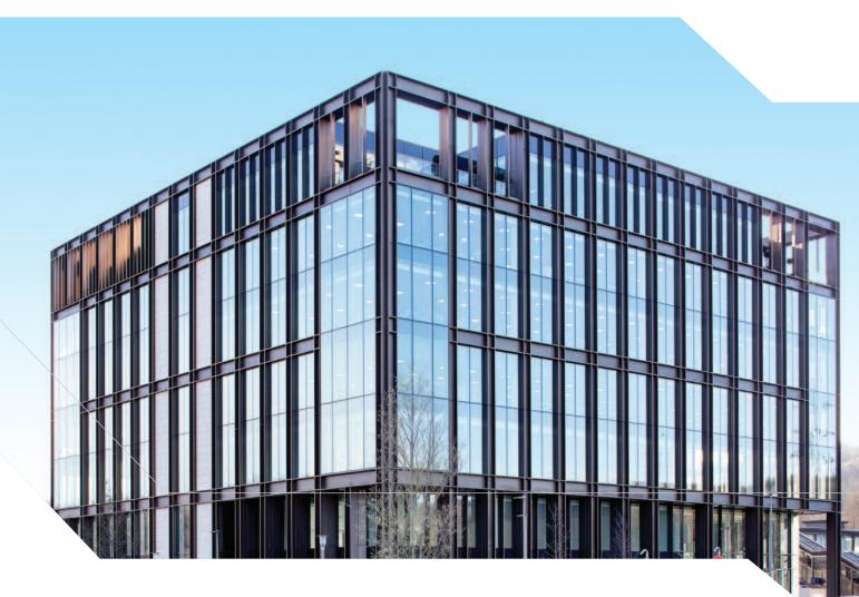
A glazed façade with deep mullions and bronze pressed aluminium panel cladding, designed, specified and installed by GLASSOLUTIONS, helped to create the ideal balance between aesthetics and functionality at Number One Kirkstall Forge, a state-of-the-art office building at the brand-new Kirkstall Forge 'urban village' in Leeds.
