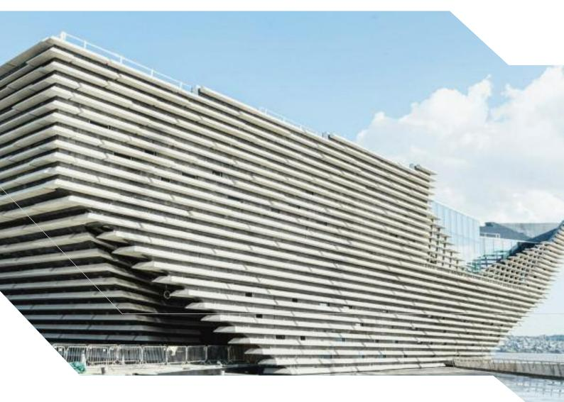
GLASSOLUTIONS overcame a unique set of design and installation challenges, including water pressure and wave loading, to install the flagship VS-1 curtain walling system at an iconic new addition to the Dundee waterfront: The V&A Museum on the banks of the River Tay.
