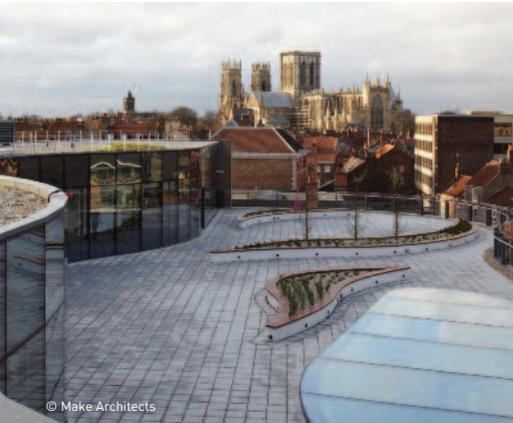
The installation at The Hiscox Building in York features Wicona curtain walling to the punch hole windows and louvres, roof terrace curtain wall, a bespoke structurally bonded rooflight and GLASSOLUTIONS' patented VS-1 glazing system to form the main atria screen and terrace parapet.
