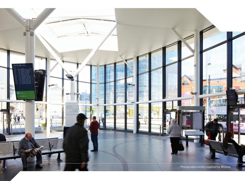
Glazing for the internal and external façades and shop frontages for the Rochdale Transport Interchange was designed by GLASSOLUTIONS to create a frameless, glass-to-glass appearance and achieve visual consistency across the project.
