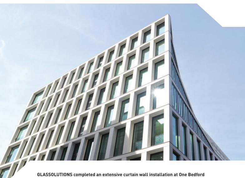
GLASSOLUTIONS completed an extensive curtain wall installation at One Bedford Avenue, a new mixed-use development in a prominent area of central London. Using an innovative, specially designed sliding track system to install the glass units, GLASSOLUTIONS was able to reduce the footprint of the site, safeguard the installation team from the risks associated with working at height, and advance the speed of the installation by a very considerable margin.
